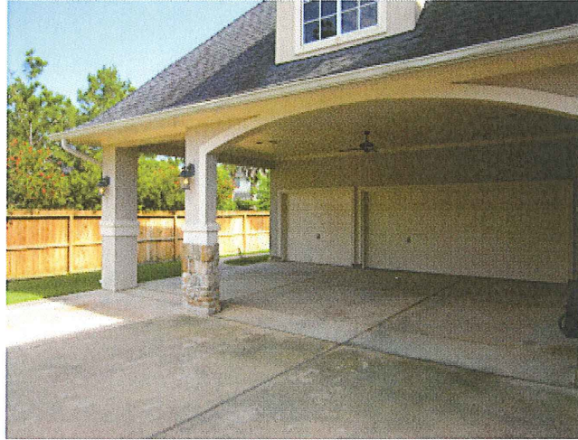
THREE CAR FRONT-LOAD GARAGE WITH PORTE-COCHÈRE Photo 1
